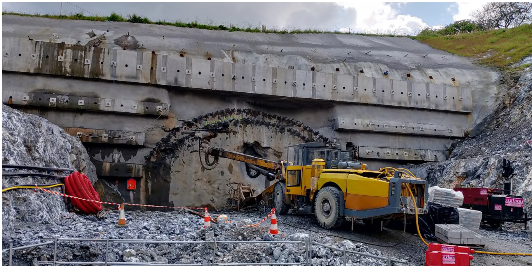
EMBOQUILLE TUNEL MARKINA
