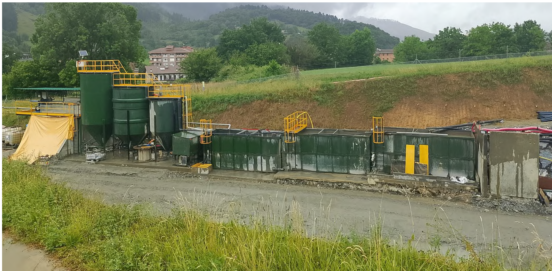
DEPURADORA EMBOQUILLE MARKINA
