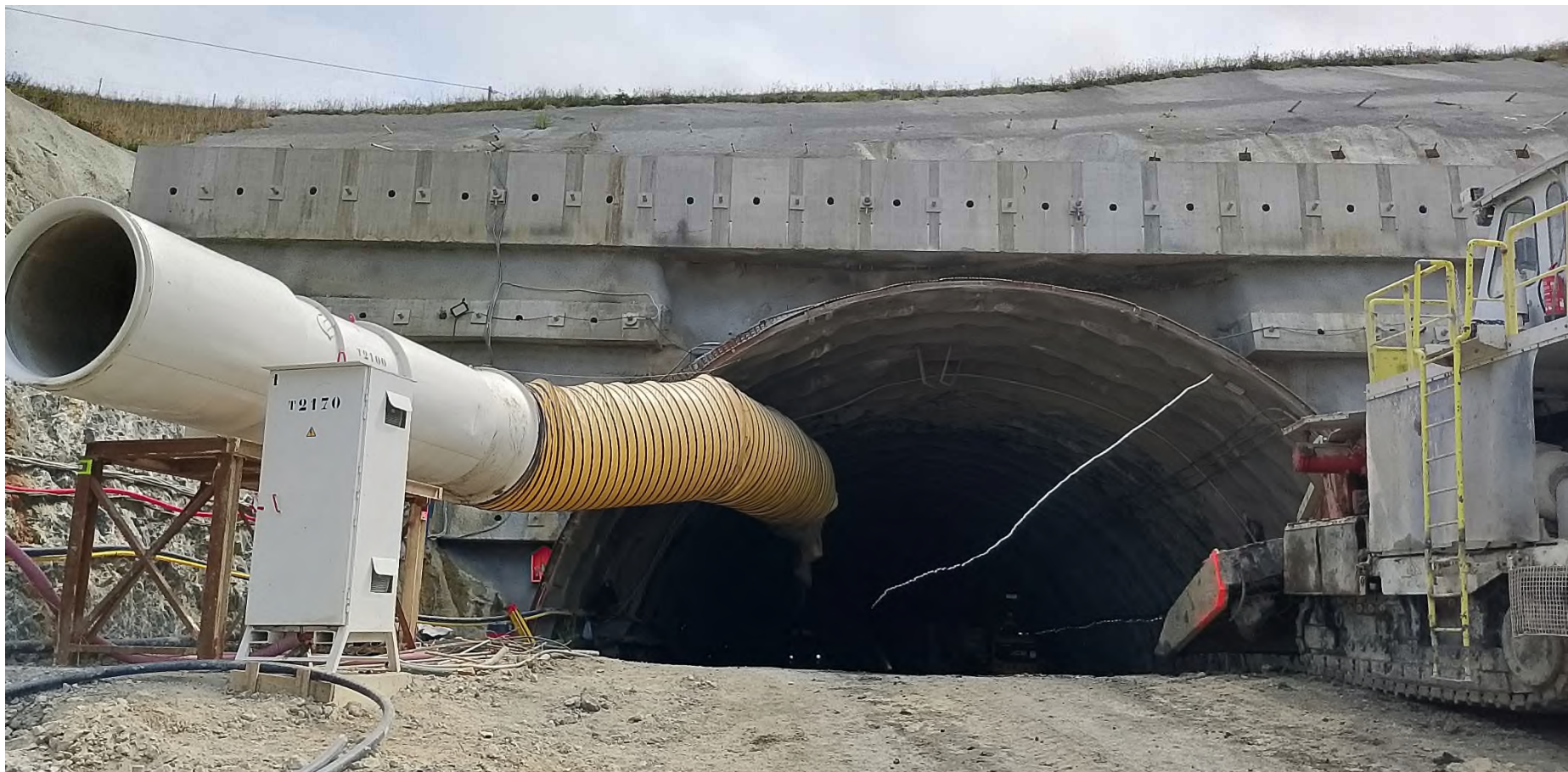
EMBOQUILLE TUNEL MARKINA
