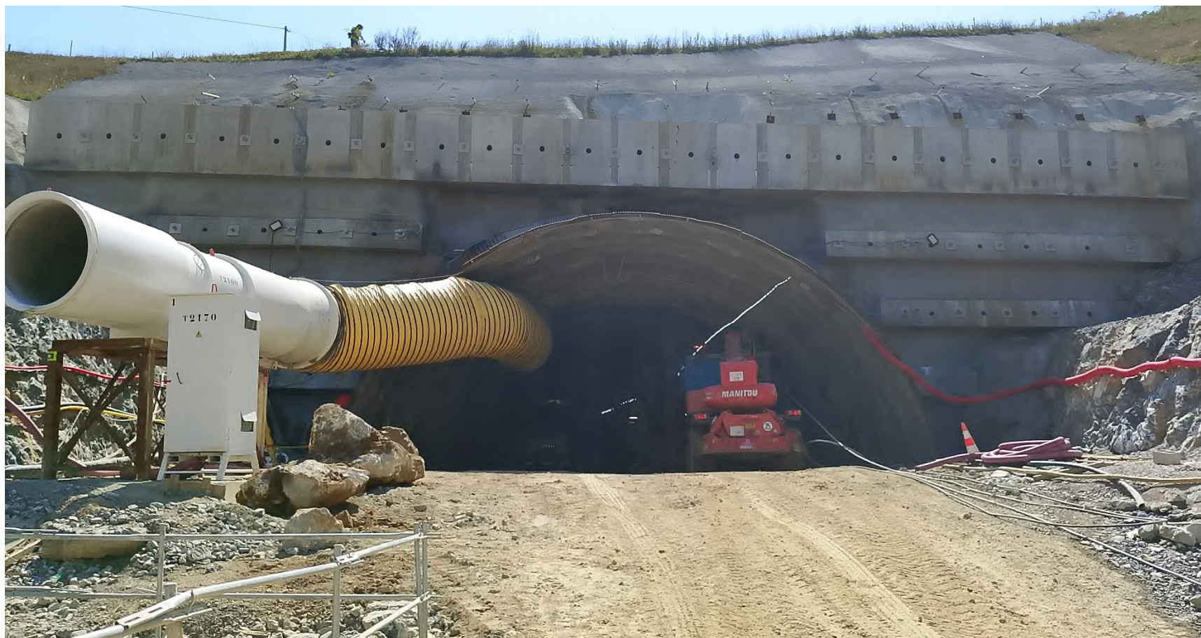
EMBOQUILLE TUNEL MARKINA
