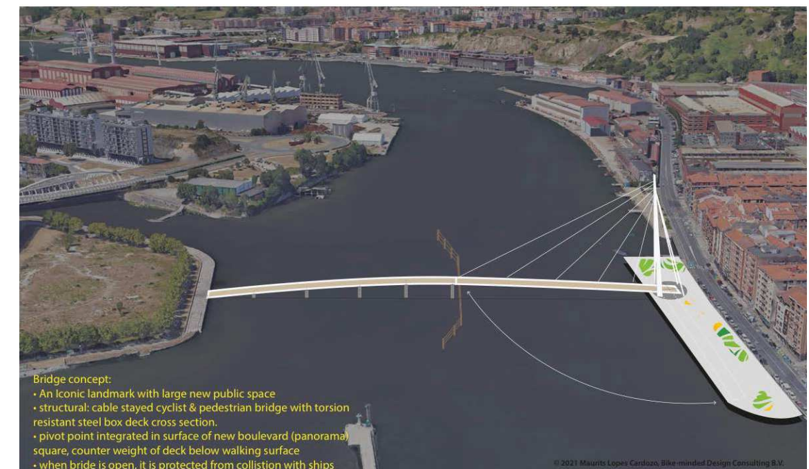
Figure 25: Alternative sketch rotating bridge including placemaking
