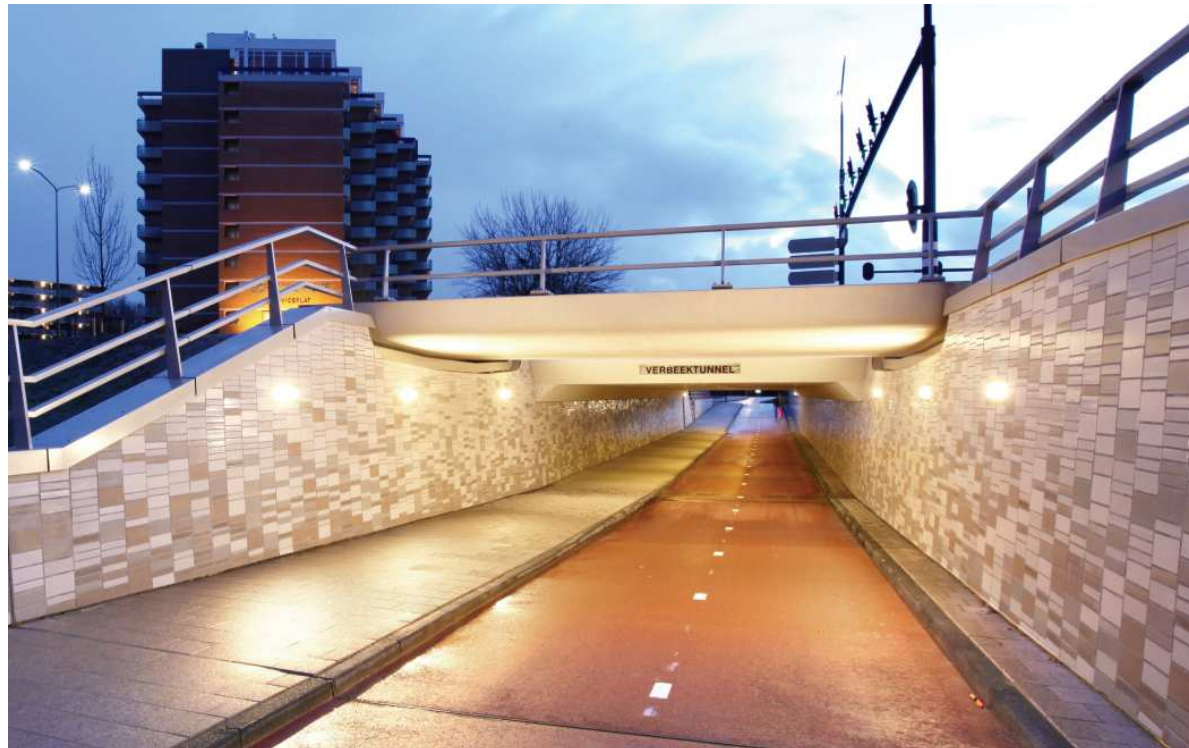
Figure 4: Example of good underpass lighting
